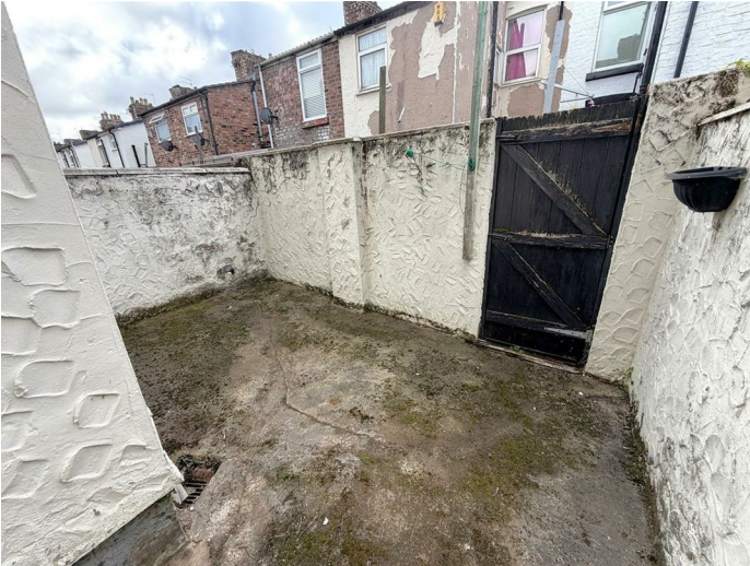
walled yard with gated access to rear
